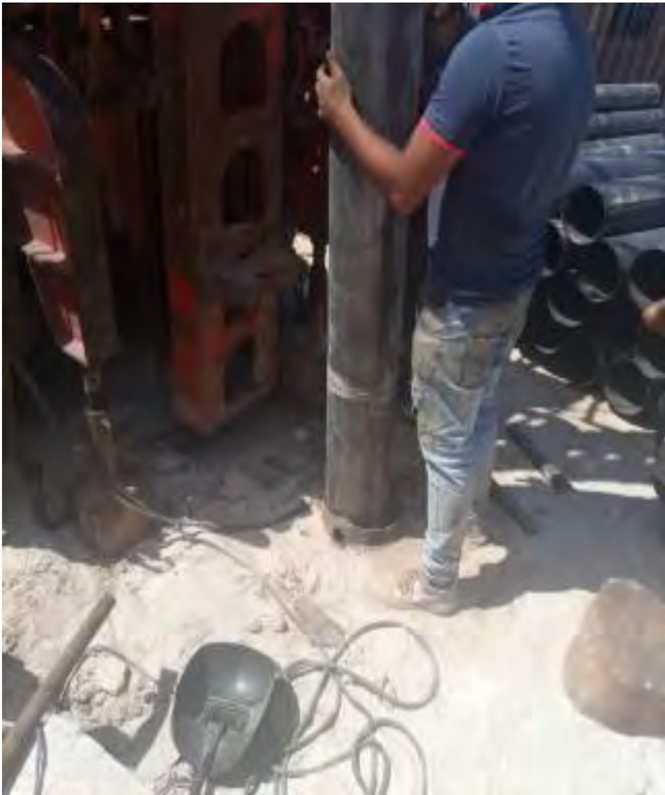
Water well pump & pipes installation
