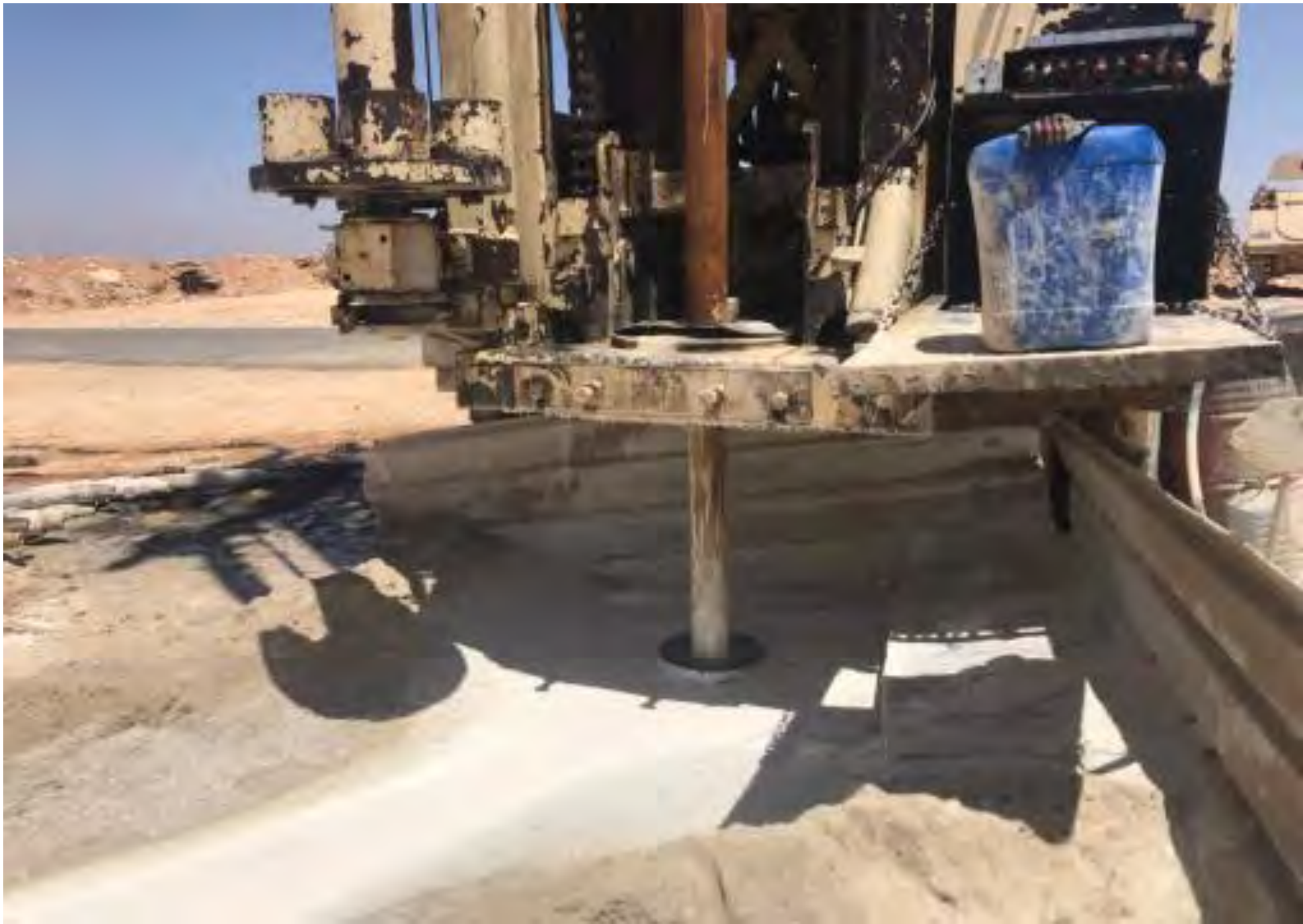
WATER WELL @677 m depth
