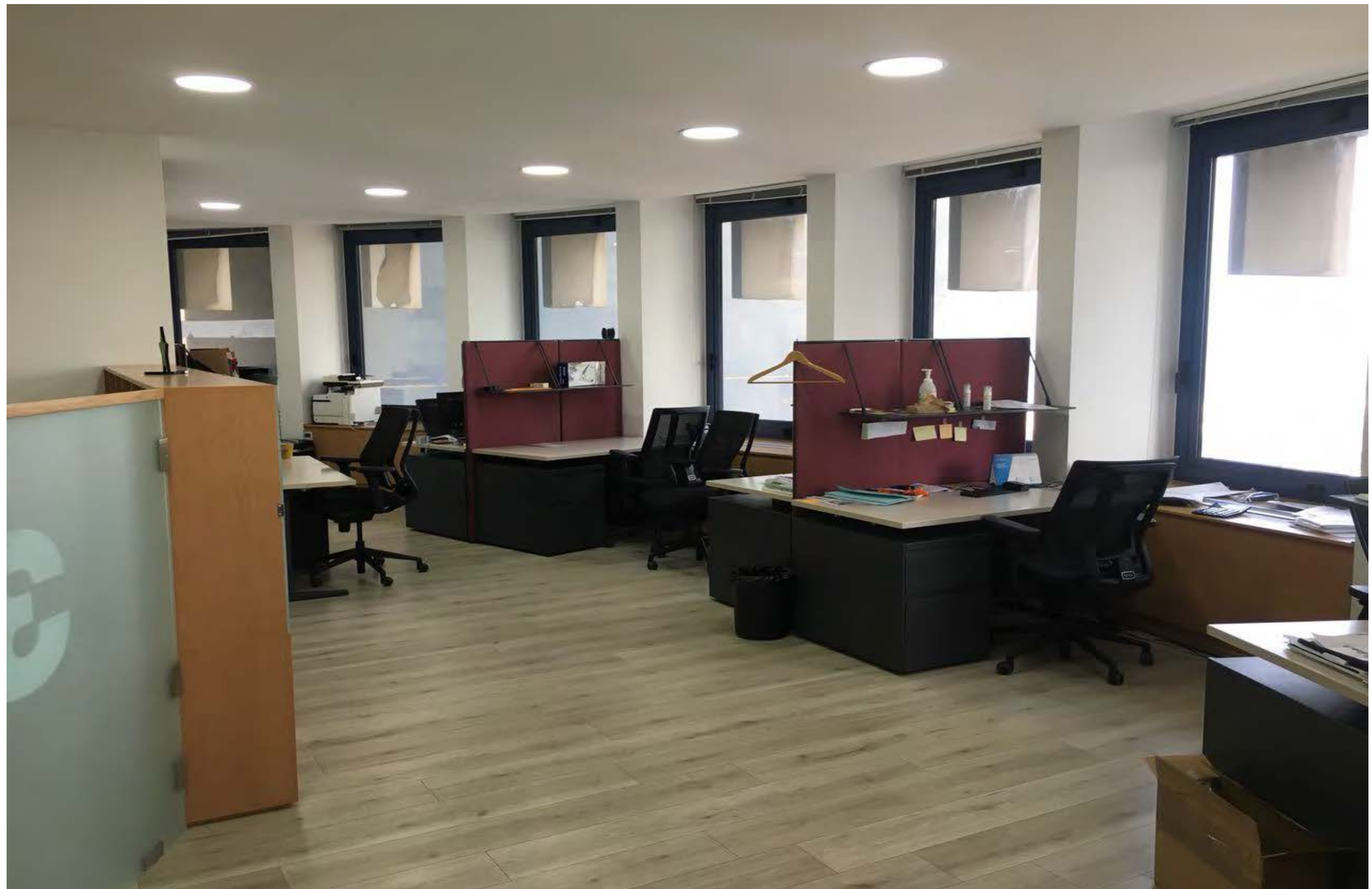
Restauration Works 200sqm 3M Head Office-St. Charles Building Mina EL Hosn (January 2017)
