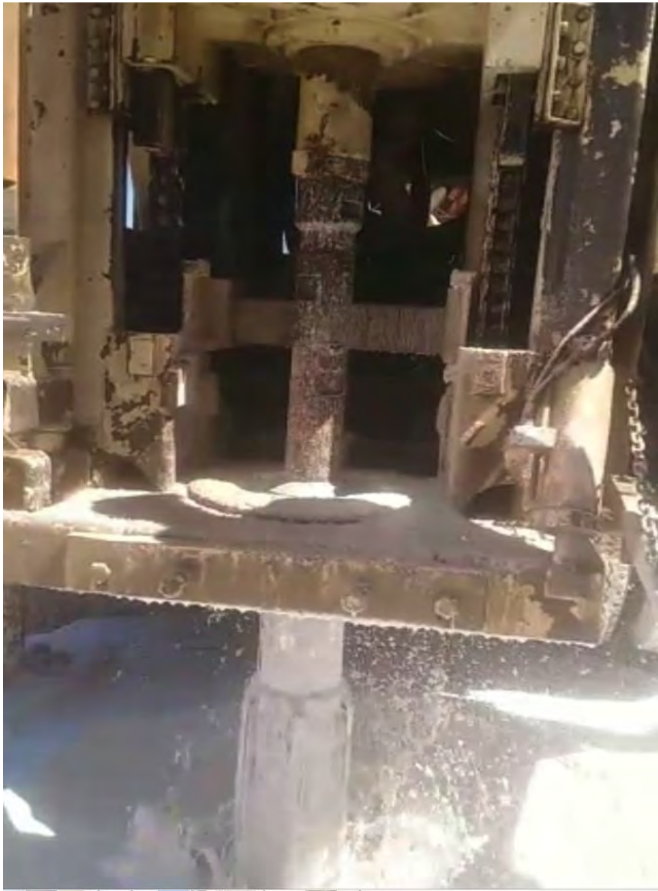
WATER WELL @ 600 m depth
