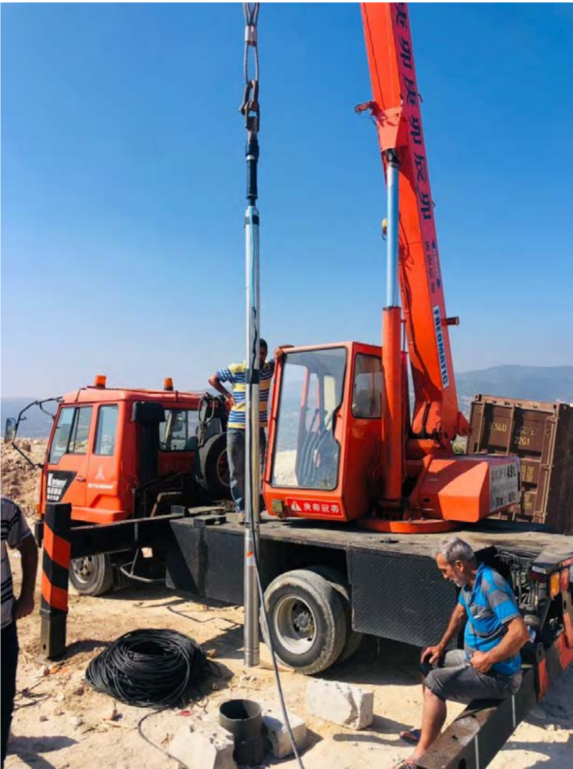
WATER WELL @ 441 m depth
