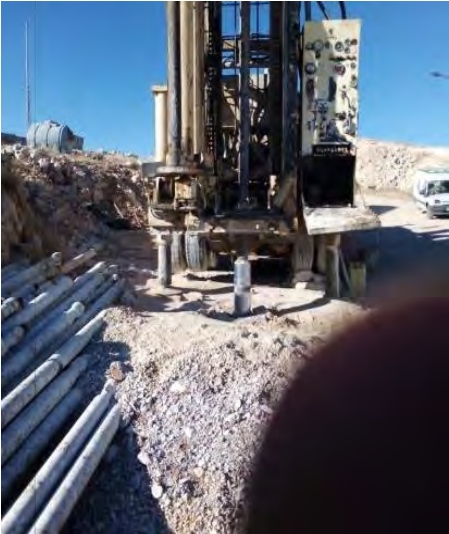
WATER WELL @ 540 m depth
