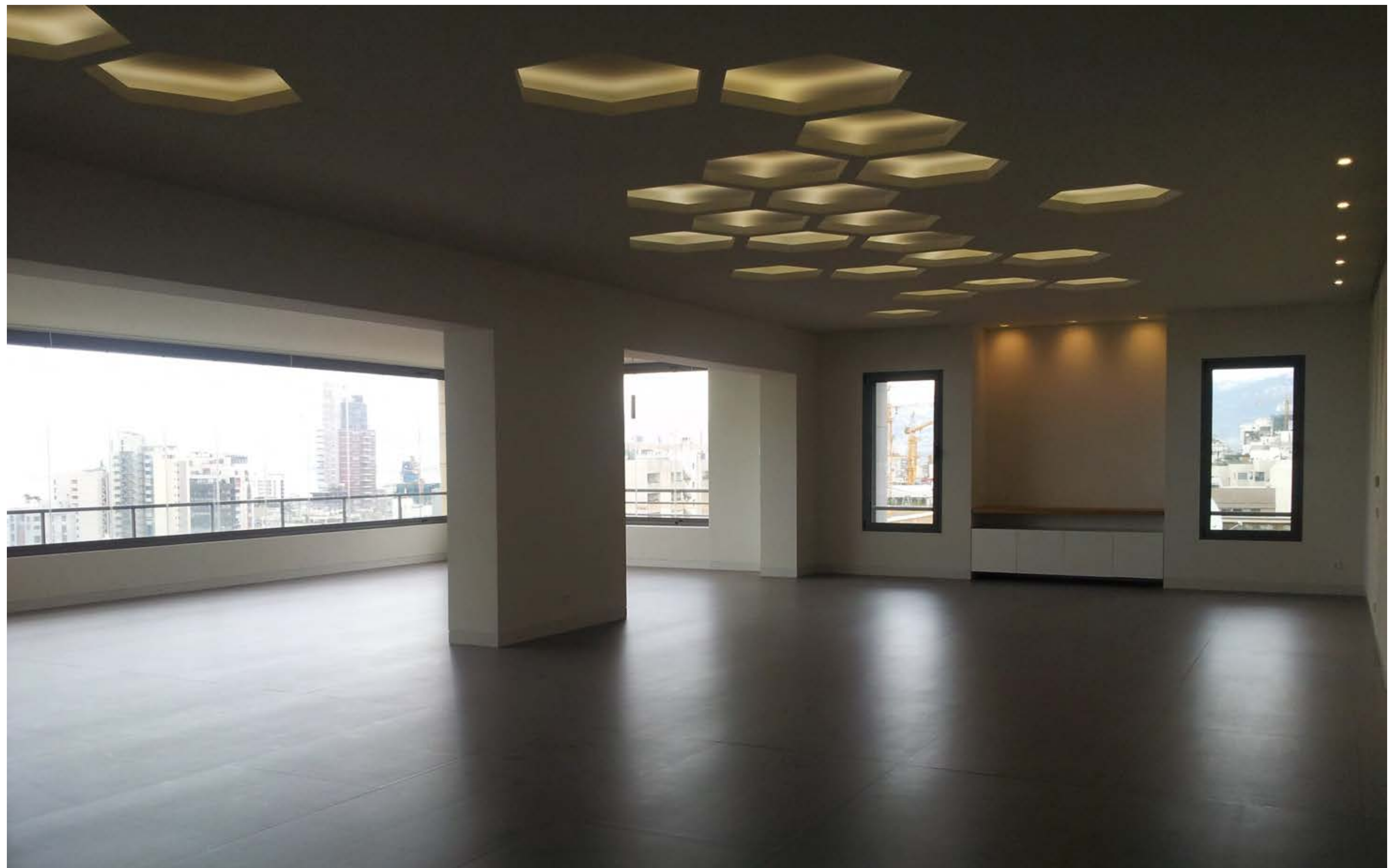
Finishing Works 550sqm Juliana Khalaf apartment-Ashrafieh (2011)
